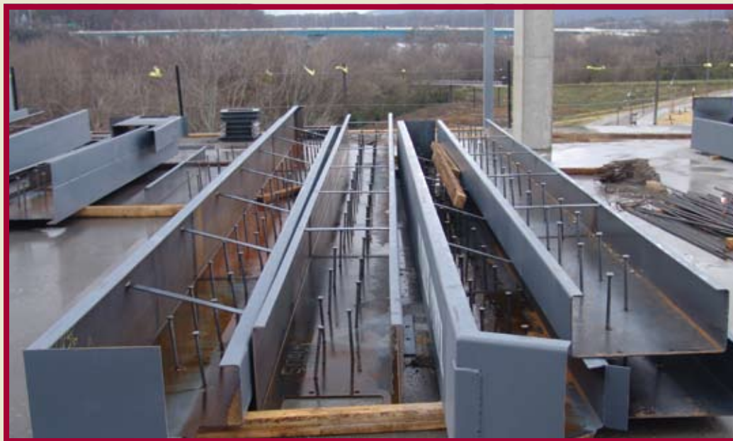
Several of the VERSA:T: beams, both interior and exterior. The composite nature of the beam enables longer spans, allowing architects to incorporate more open floor plans into their building designs.
