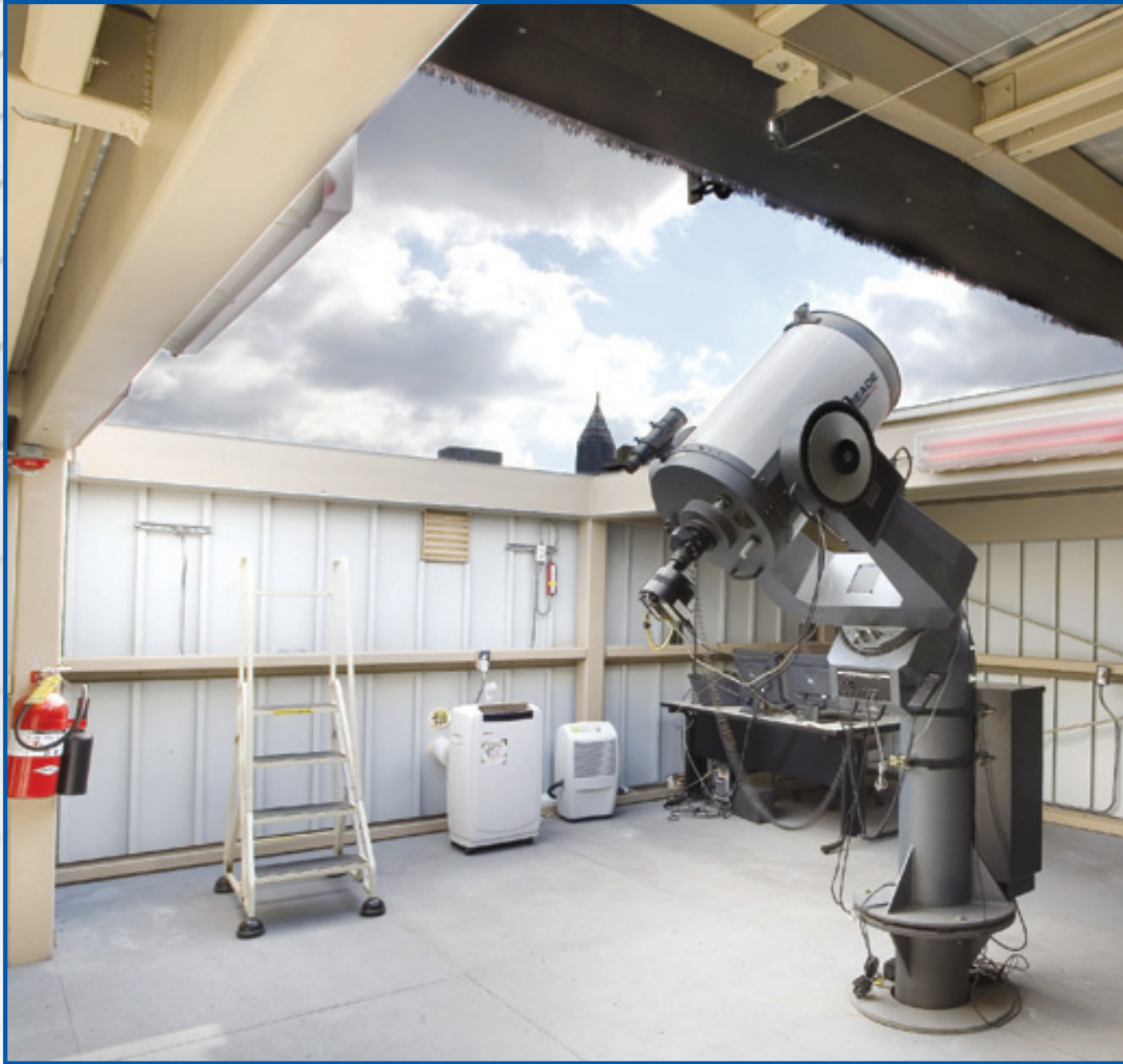
The Howey Physics Observatory at Georgia Tech was a design-build project completed in 2006. Built on top of challenges, including a fully retractable e roof. "It was an interesting task," explains Doug Beatty, "as we had to
