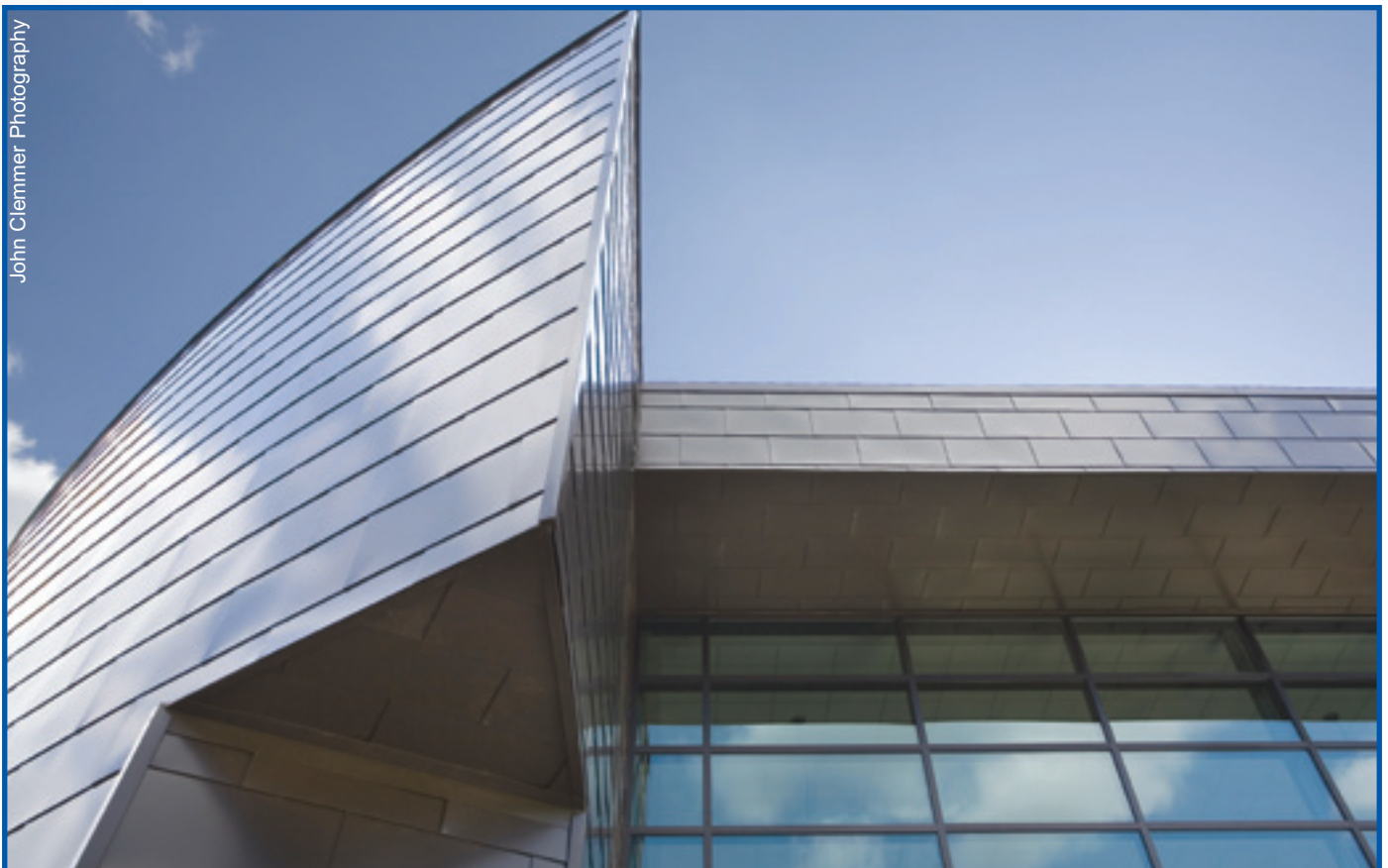
The outer shell of the Success Center is made of Kynartm-painted interlocking steel panels. The placement of the panels had to be exact to conform to the architectural design of the building.
