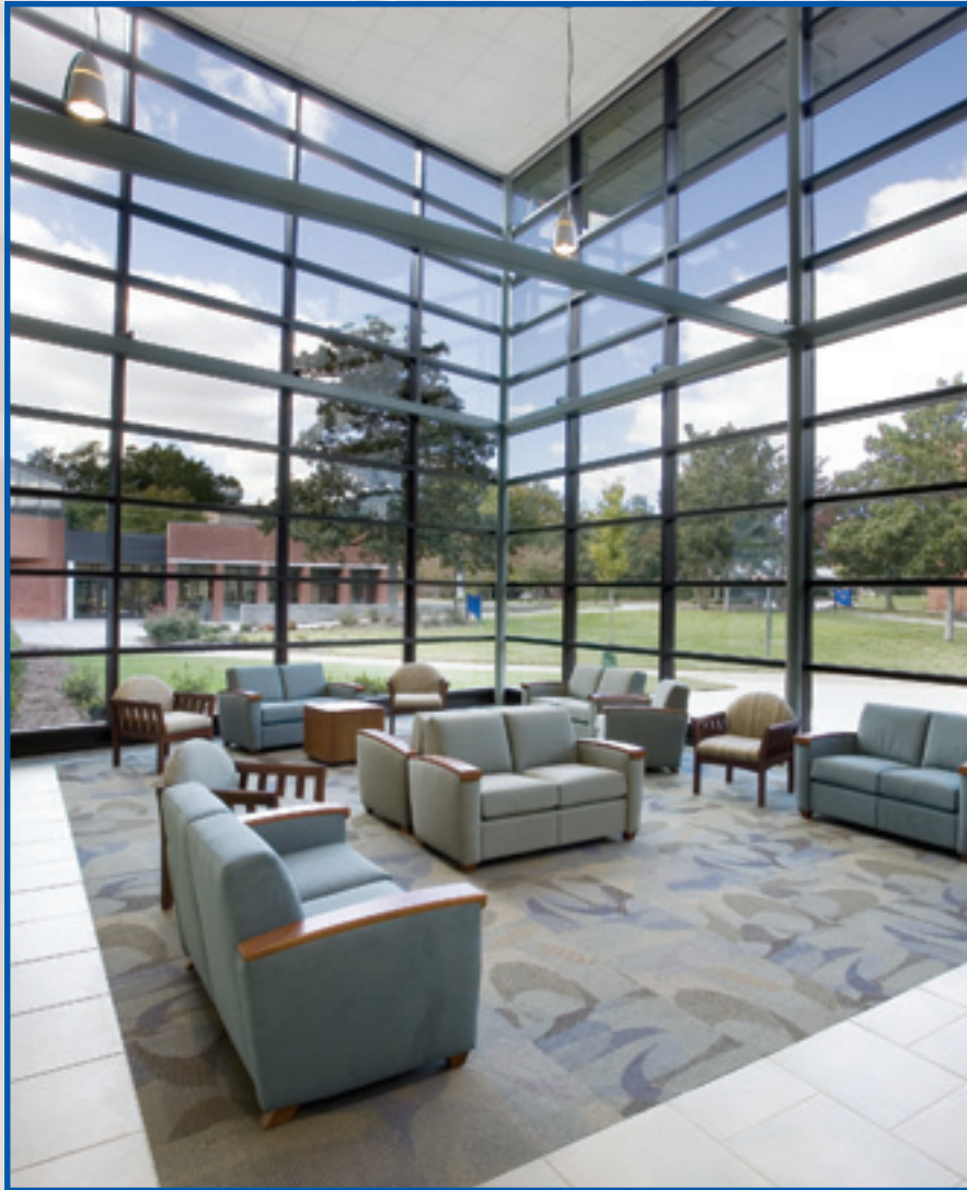
Inside the Gordon College Success Center, looking out towards the campus. The curtainwall windows needed an extra brace to withstand the potential wind load against it, another example of the “hand-in-glove” philosophy that Beatty Construction embraces. “We work directly with the architects and engineers to make sure that the customer gets what they want. We’ll find a way to make it work,” says Beatty.
